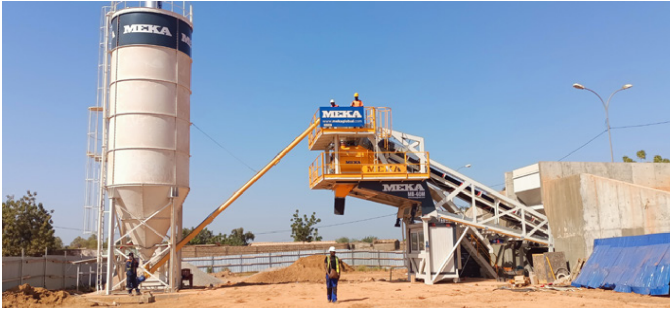
▲ Meka Mobil Beton Santrali Kurulumu-2024 Burkina Faso
