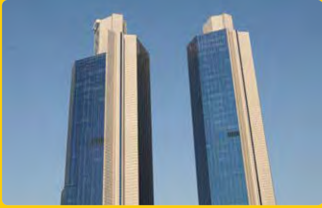
Sabancı Center – İstanbul, 1991
